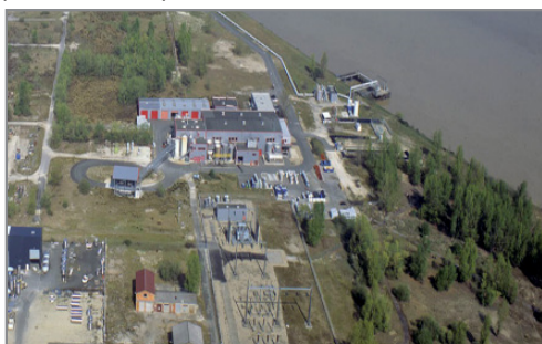
View of production plant in Ambès, France.
